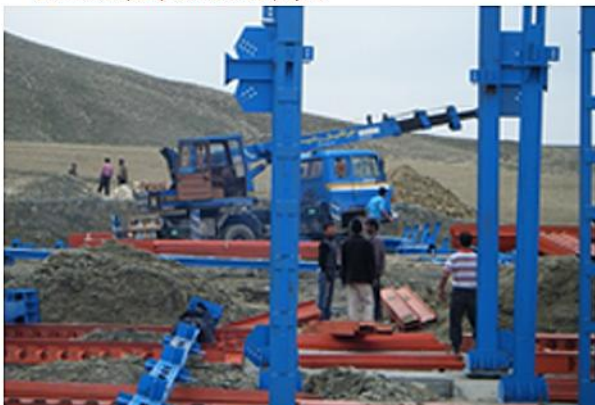
▲ Construction supervision of Tekab Housing Cooperation project
