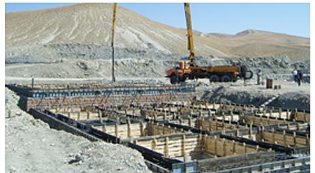
▲ Construction supervision of Mehr Ghadir project
