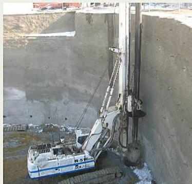
▲ Pile Installation, Tavrij Residential Tower
