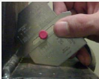
▲ Welding quality control
