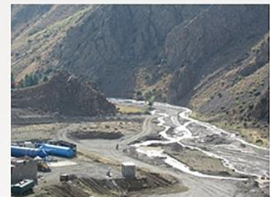
▲ Quality control of Earthwork operations
