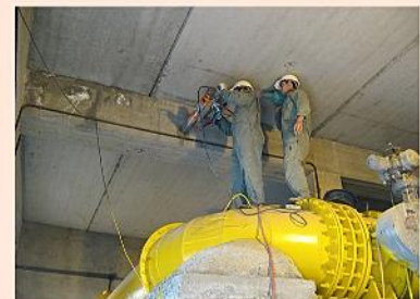
▲ Z.J Engineering technician using coring machine
