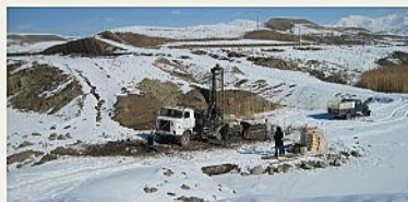
▲ Exploration drilling, Spiran bridge site
