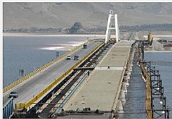
▲ Quality control of Asphalt implementation of Urmia lake's bridge
