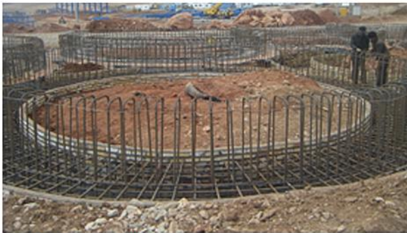
▲ Concrete quality control of silo project
